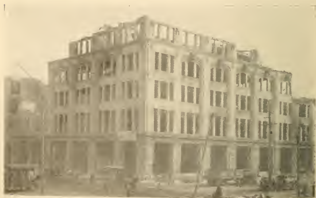
General View of Building at First and Mission
